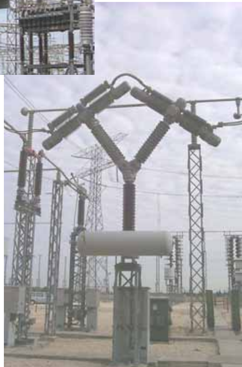
High speed bypass breaker across the converter on the dc side.
