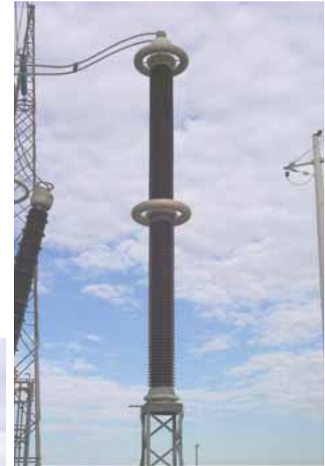
DC side Voltage Divider
