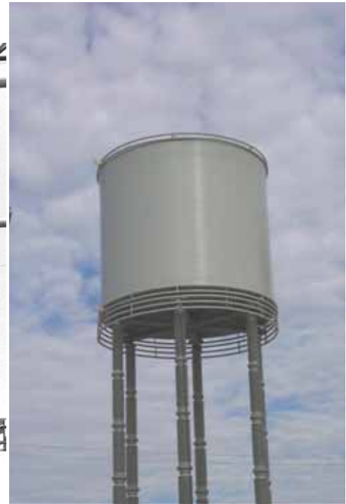
New style air-cored smoothing reactor
