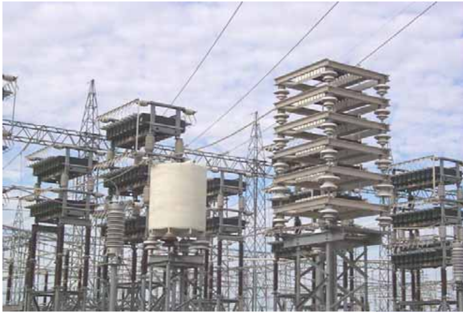
AC High pass filter. Being a HP filter no seasonal tuning is necessary. However the filter has a resistor in parallel with the reactor (the rectangular tower on the right)
