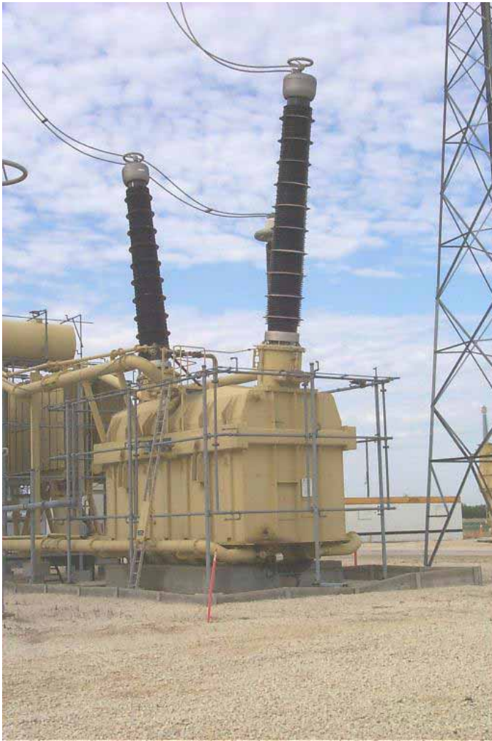
Older style oil-coiled smoothing reactor in tank
