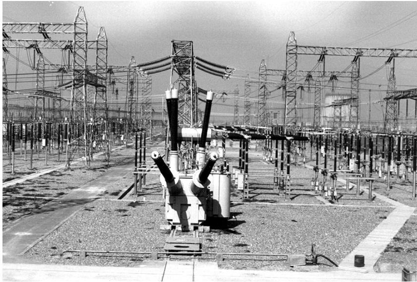
Spare Converter Transformer in switchyard (Dadri, India)
