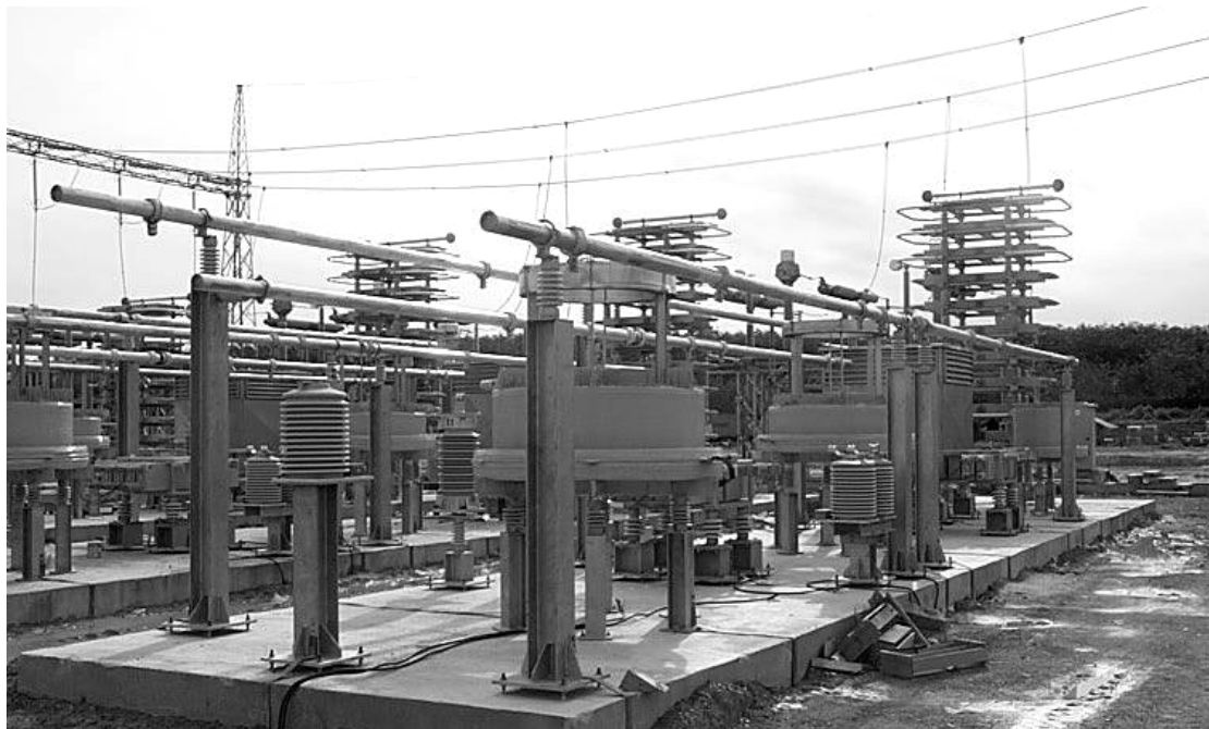
Air cored smoothing reactor
