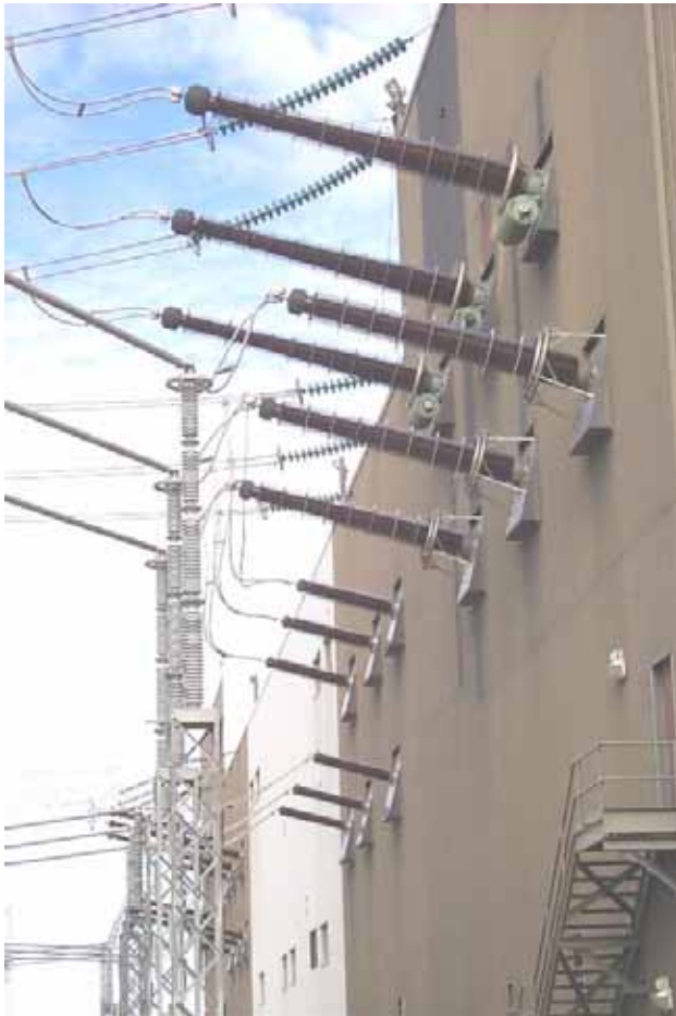
AC Side Bushings in Valve Hall
