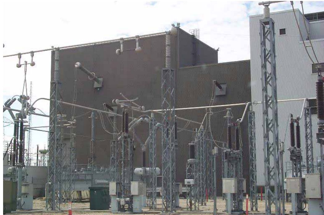
Top: DC Side Bushing in Valve Hall
