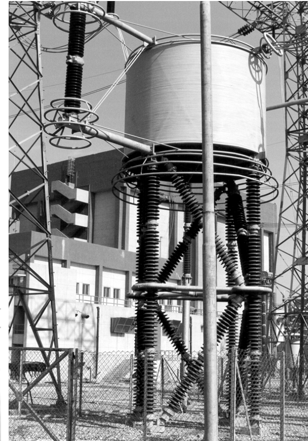
Air cored smoothing reactor
