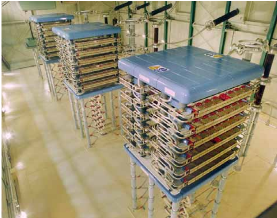
Inside of Valve Hall and Quadri-Valves
